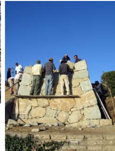
LEFT: TETSU SPLITTING STONE WITH TOBI-YA CHISELS. MIDDLE: DONNA HASBROUCK, A MASON FROM LOPEZ ISLAND, CUSTOM CUTS A FILLER STONE. RIGHT: THE CREW AT WORK. NOTE THE WHITE TOBI-YA CHISEL MARKS.
