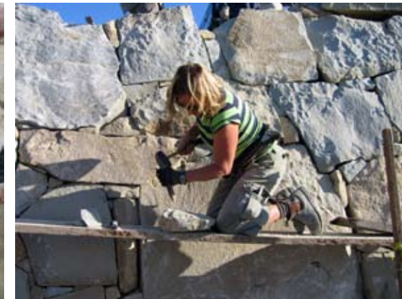
LEFT: TETSU SPLITTING STONE WITH TOBI-YA CHISELS. MIDDLE: DONNA HASBROUCK, A MASON FROM LOPEZ ISLAND, CUSTOM CUTS A FILLER STONE. RIGHT: THE CREW AT WORK. NOTE THE WHITE TOBI-YA CHISEL MARKS.
