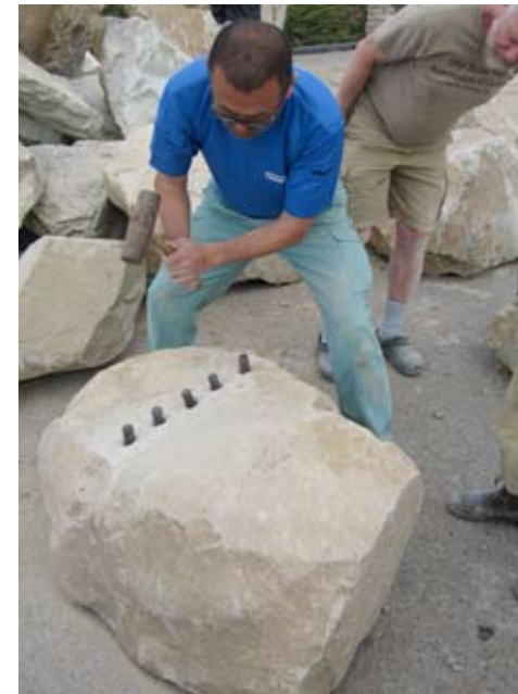
LEFT: TETSU SPLITTING STONE WITH TOBI-YA CHISELS. MIDDLE: DONNA HASBROUCK, A MASON FROM LOPEZ ISLAND, CUSTOM CUTS A FILLER STONE. RIGHT: THE CREW AT WORK. NOTE THE WHITE TOBI-YA CHISEL MARKS.
