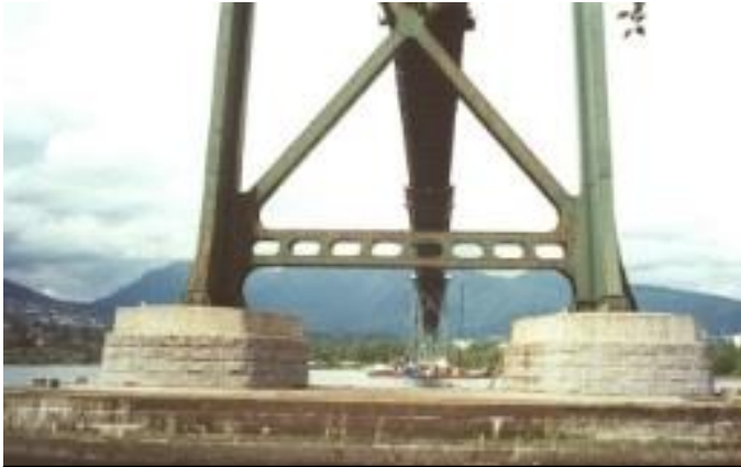
Lion's Gate Bridge Footings Vancouver B.C.
